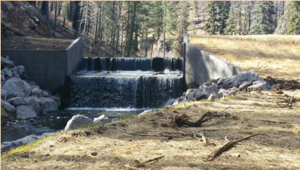
Willow Creek fish barrier, Catron County, New Mexico protects the resident Gila Trout population from encroachment of non-native trout.
